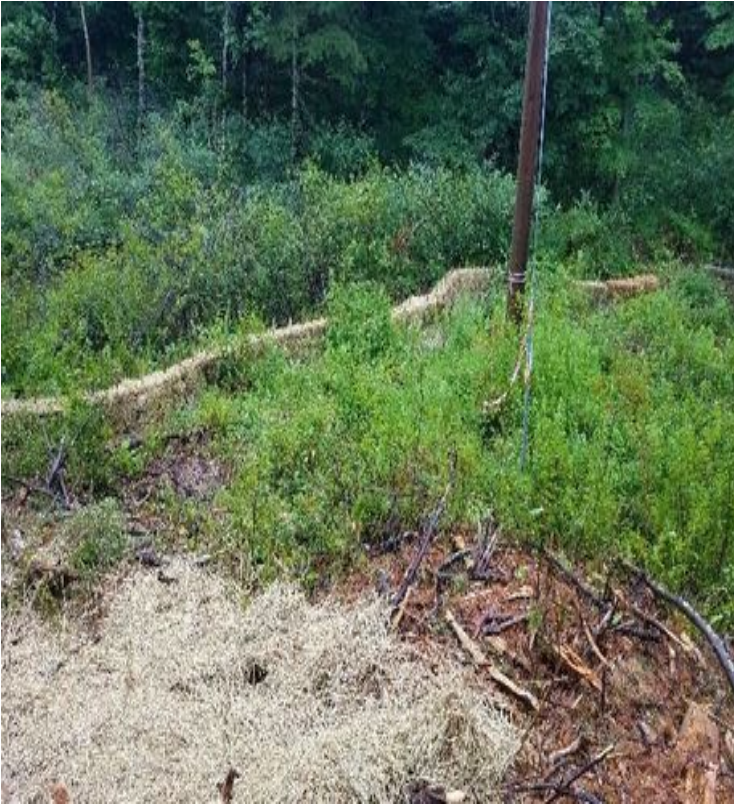
Fig 13: Straw bales installed between Str.28 and Oyster River. Viewing north. (7-23-19).
