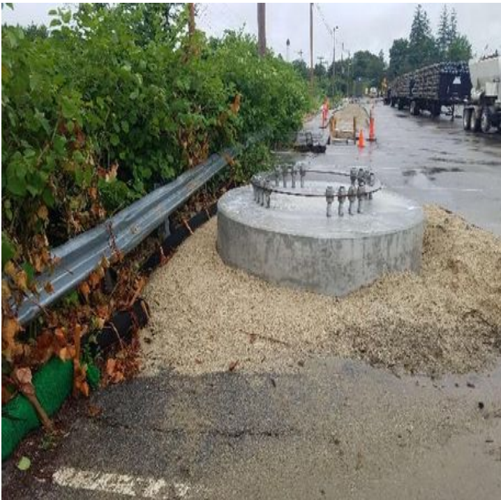
Fig 11: Filter sock installed around Str. 22. Viewing south. (7-23-19).
