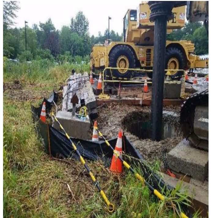
Fig 6: MJ drilling Str. 23, next to wetland DW67. Viewing west. (7-23-19).
