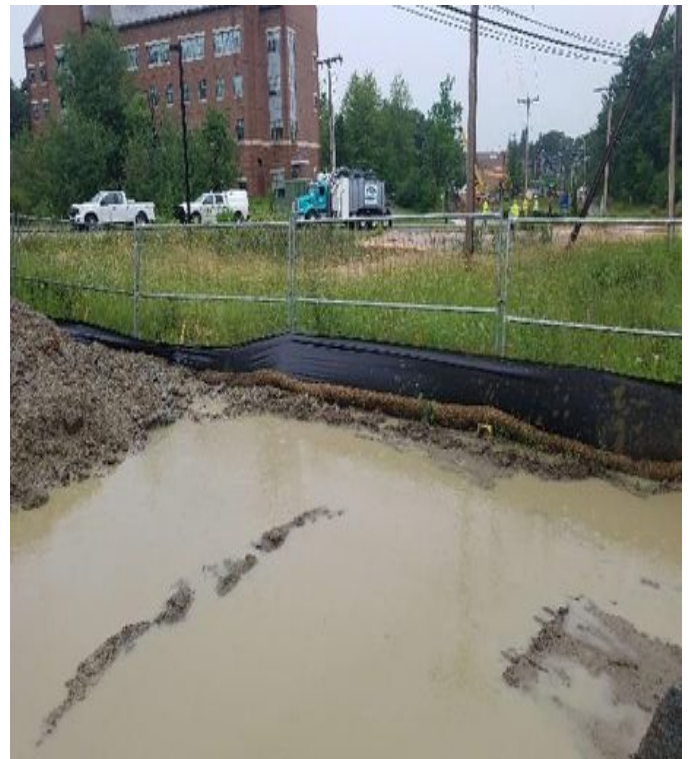
Fig 8: Area in Waterworks Rd laydown yard where straw bales are recommended. Viewing north. (7-23-19).
